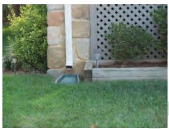
Figure 4.32. Rooftop disconnection (photo: Center for Watershed Protection, Inc.)
