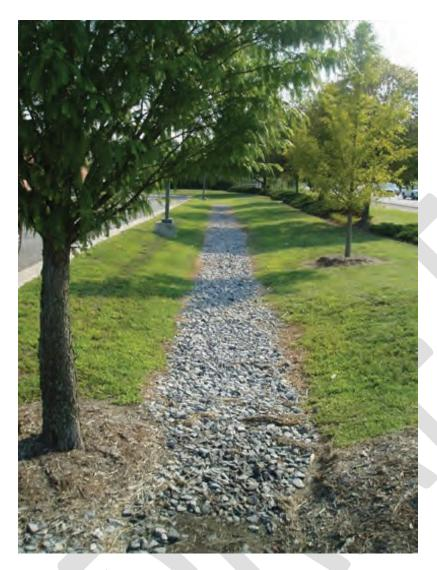
Figure 4.16. Infiltration practice in median strip.
