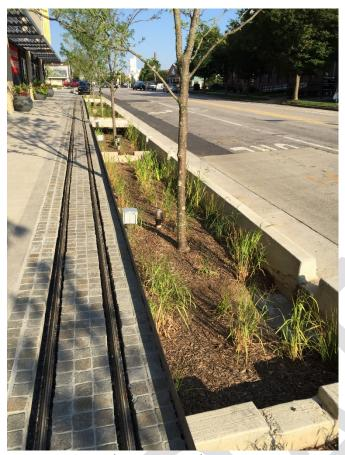
Figure 4.5. Example streetscape bioretention.
